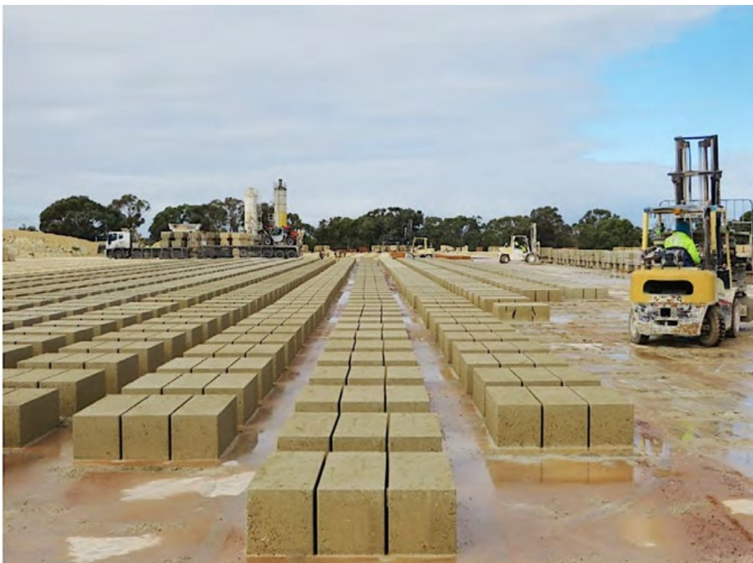
Figure 3: Block making plant
